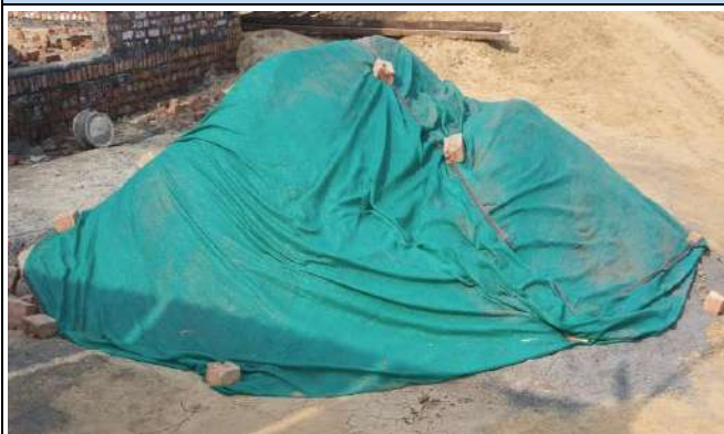
COVERED CONSTRUCTION MATERIALS
